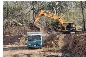
Excavation and Backfill Zone 1
