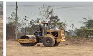
Soil grading and compaction zone 2
