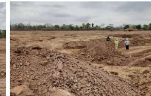
Backfill the pond Zone 3
