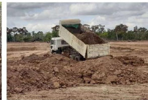
Backfill and Grading Zone 1
