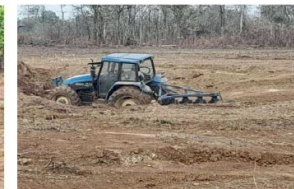
Backfill and Grading Zone 3
